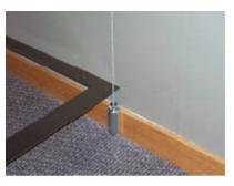
4. Using the square as a guide, draw a 3 " long line on the floor starting from 16 3/8" (extending to 19 3/8"). Repeat on the other side of the wall mounting plate. The floor mounting plate is located between these two lines. If the Wall System is being installed using a 2" x 6" external backer board, the line will start at 17 7/8" and extend to 20 7/8".
