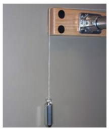
3. Drop a plumb line down from one end of the wall mounting plate. Place the framing square so that one leg is along and one leg is perpendicular to the wall. The leg that is perpendicular to the wall should be placed against the plumb line (see next photo).
